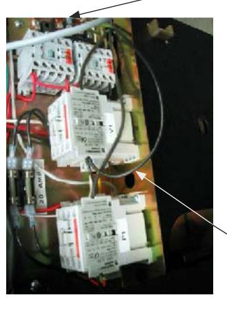
Connect black wire from heater to contactor V1 terminal L1 as shown
