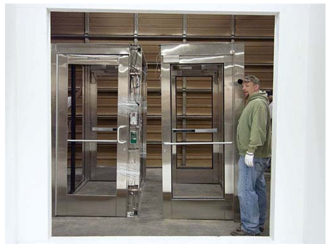
Vestibule halves as viewed through the rough opening
