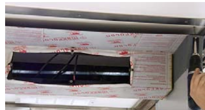
Installing the metal detector bridge
