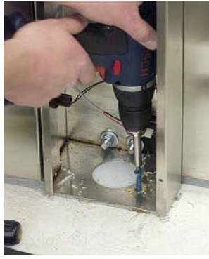
Anchoring rear center post
