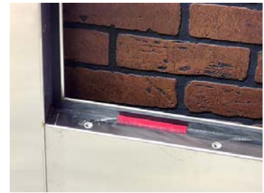
Positioning glass blocks
