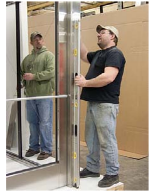
Leveling the assembly
