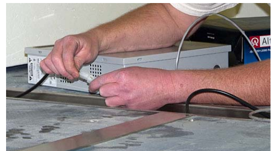
Installing the power supply
