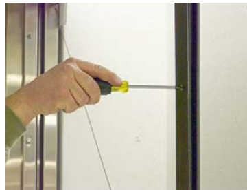
Installing center mullion
