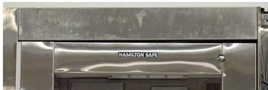
Poor door gap
