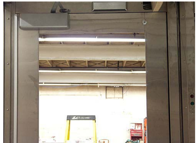
Good door gap
