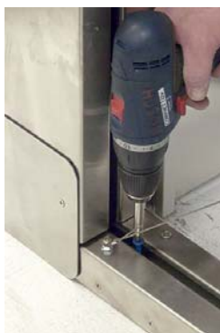
Anchoring bottom rail
