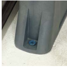
Attaching panels to floor
