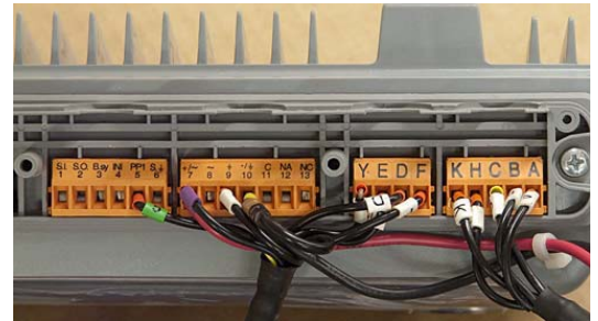
Attaching cables to control panel
