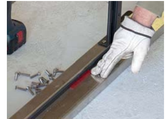
Positioning glass blocks
