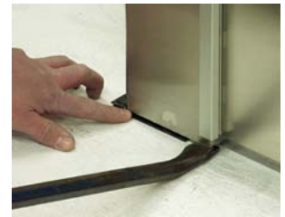
Installing non-metallic shims
