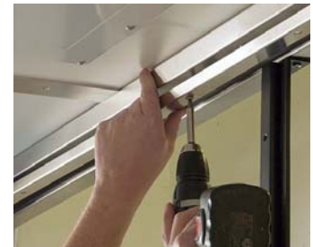
Installing top horizontal glass channel
